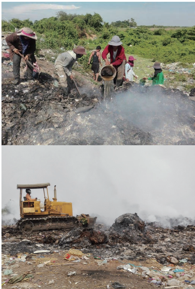
Figure 13: Extinguishing Landfill Fire using Water and Soil
