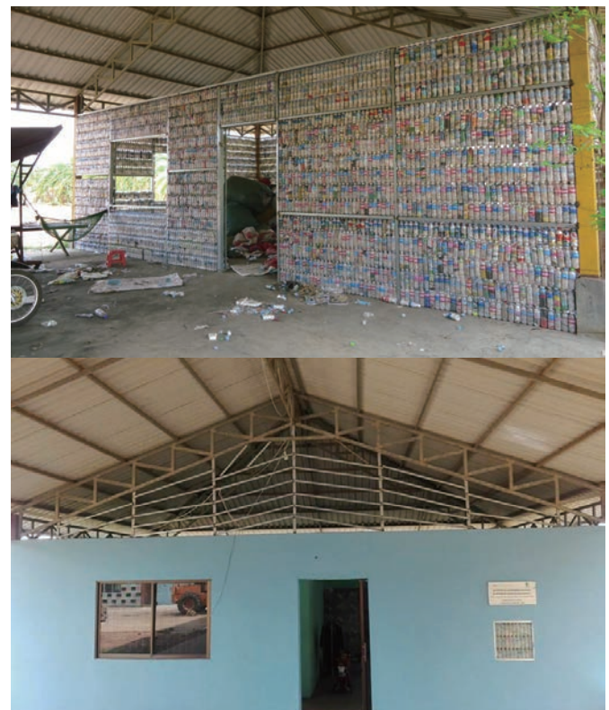
Figure 8: Use of Plastic Bottle Bricks for Construction at the Composting Centre
