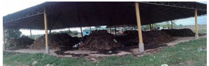
Figure 7: Composting Plant Operated by COMPED
