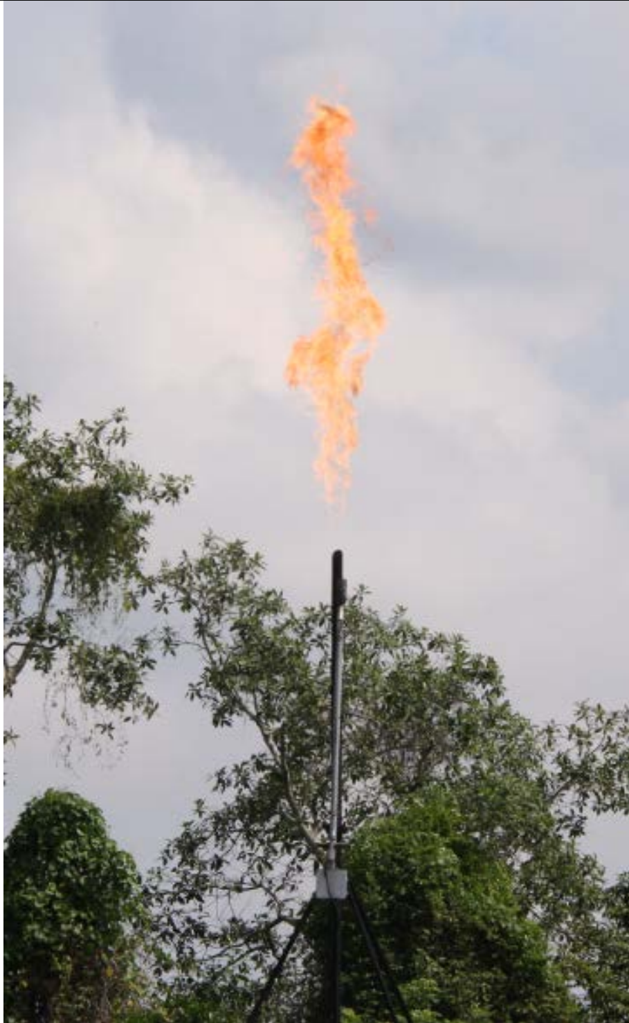
Figure 2: Photograph of the flare at the CCAC.3 Oil Battery, 8 October 2014.
