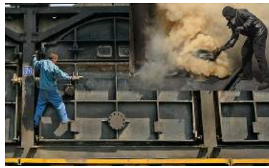
modern coke ovens
