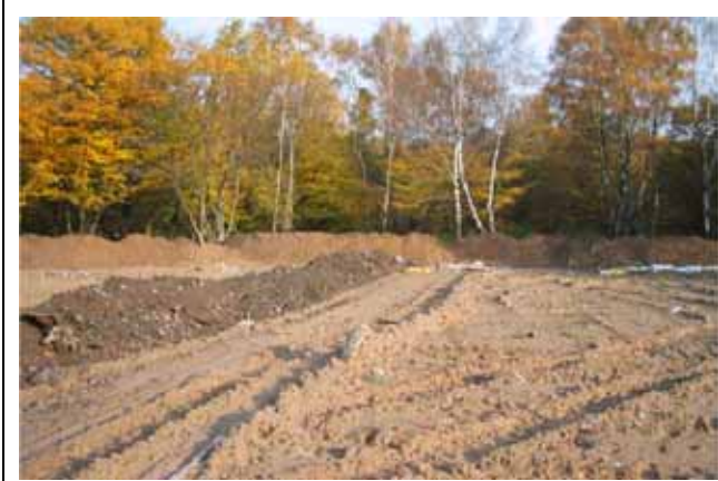
Photo 15: External bund wall together with central tipping cell bund wall.
