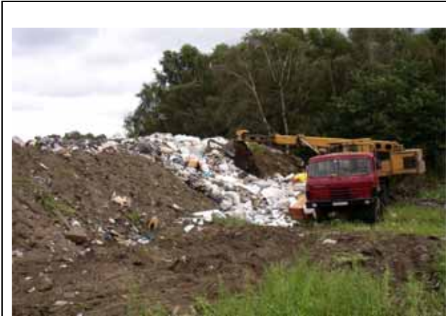
Photo 13: Construction and Tidying-Up of the bund wall on the far SW of the site.
