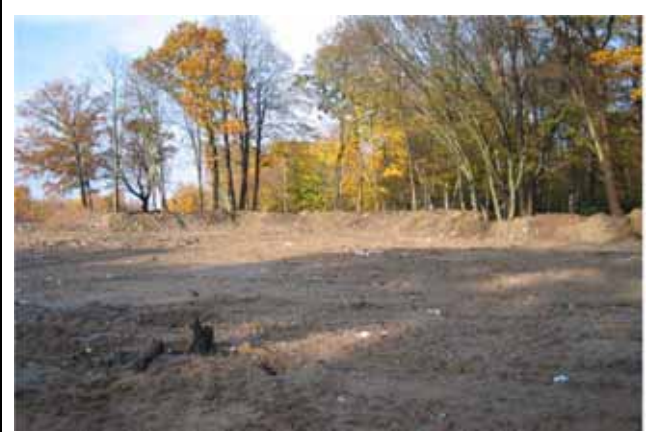
Photo 16: Completed bund wall on the NE site.
