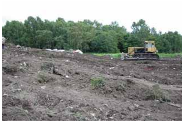
Photo 6: Process of forming the bund wall at the western edge of the site in order to regulate and consolidate the site's footprint.
