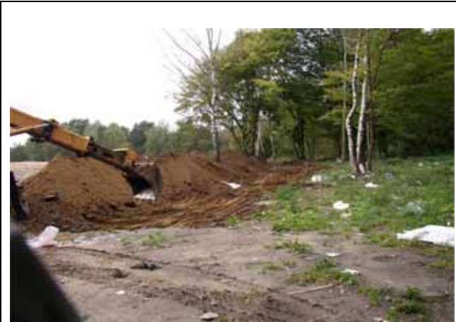
Photo 14: Construction of the bund wall on the NE perimeter of the site.
