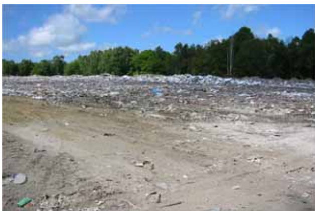
Photo 5: Process of compacting, shaping, and doming the site prior to being covered.
