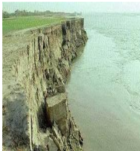
River bank erosion
