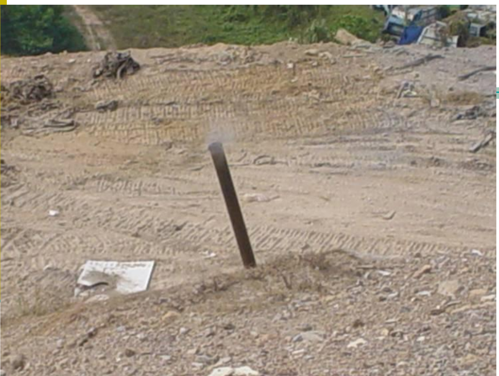
Passive release of landfill gas into the atmosphere
