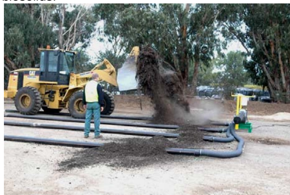
Establishing a mobile aerated floor (MAF) composting pile
