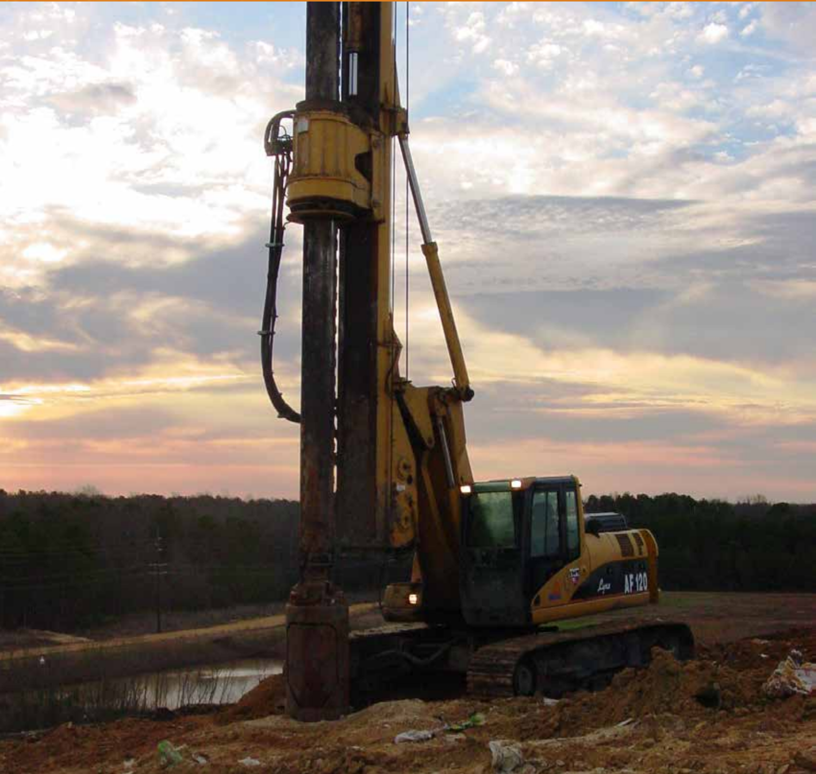
Drilling to install vertical LFG wells at an existing landfill.
