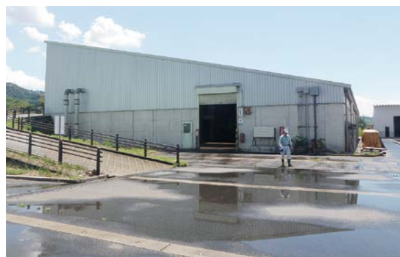
Fig. 41 Composting plant in Nagai City, Japan
