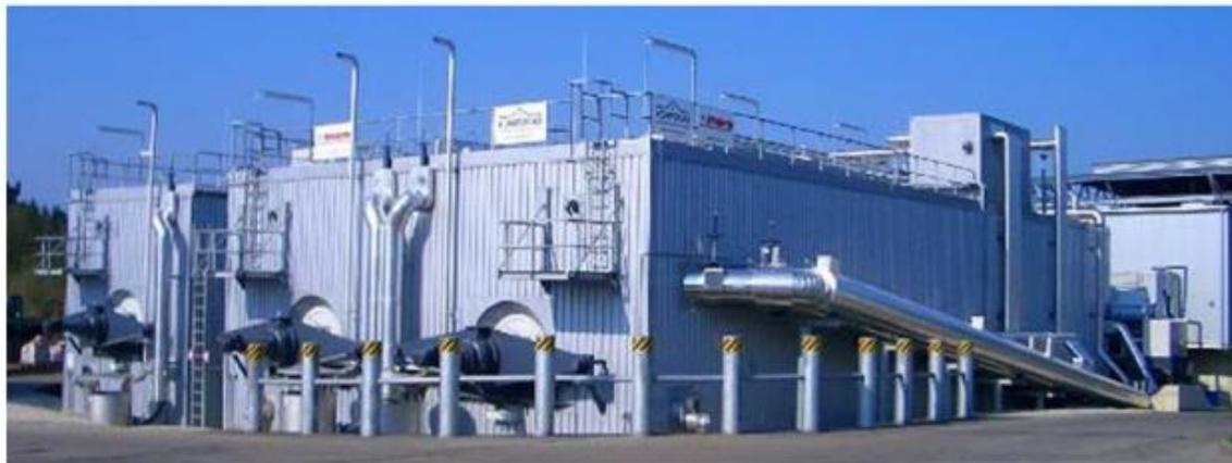
Annex I - Fig. 2: Horizontal, dry digestion system (Source: Kompogas)
