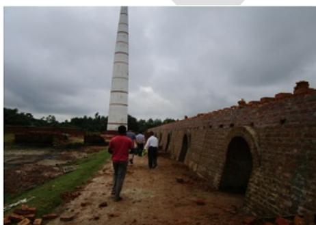
Bhatta’. It is elliptically shaped with well insulated permanent side walls and roofs and arched firing chambers that allow easy air flow. The kiln is versatile in size ranging from 22 to 42 chambers.
