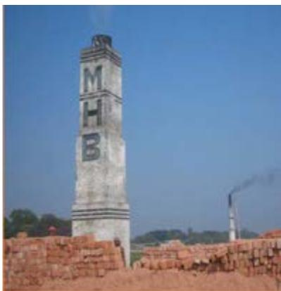
blower, which draws the flue gas from the kiln and discharges it to the atmosphere. The kiln is divided into 44 to 52 chambers, which are separated from each other in such a way that the hot gases move in zigzag path through the kiln. While some utilize a natural draft, others use a fan to draw the fire and heat through the zig-zag stacking pattern. This firing process requires a set of highly trained and skilled workers to
